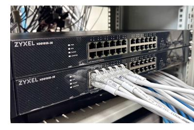
To extend connectivity and power across the building, four GS1915-8EP PoE switches were installed. By redirecting the access points to these locations, the Zyxel Networks' team streamlined the management of the wireless system and eliminated the need for separate power supplies.
